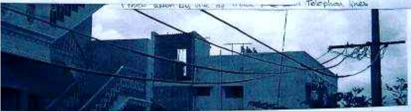
Wires Cement poles
